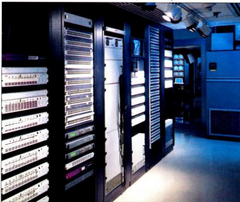
Rack room showing distribution amps, patch panels and a Liebert computer room air conditioning unit in the background.
